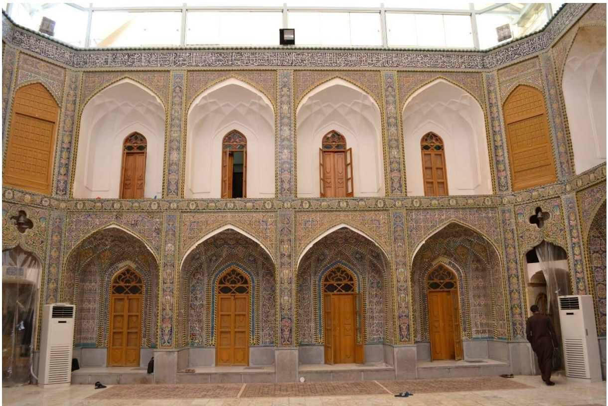
Figure 207: La façade Nord de la cour de la Madrasa al-Sayyid Muhammad Kāzim al-Yazdī
