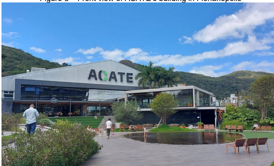
Figure 8 – Front view of ACATE's building in Florianópolis
